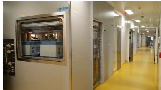
A view inside the new P3 containment lab, showing unit for drug screening (photo courtesy of Pieter Leyssens).
